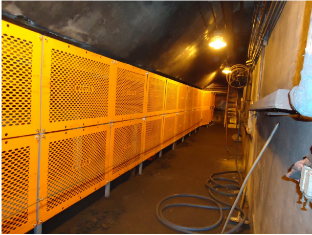
Martin Engineering installed 400 feet of guarding.
