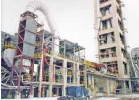
*Material buildups in the pre-heater tower at the Holcim Devils Slide Plant led to the installation of Martin® Air Cannons.*
