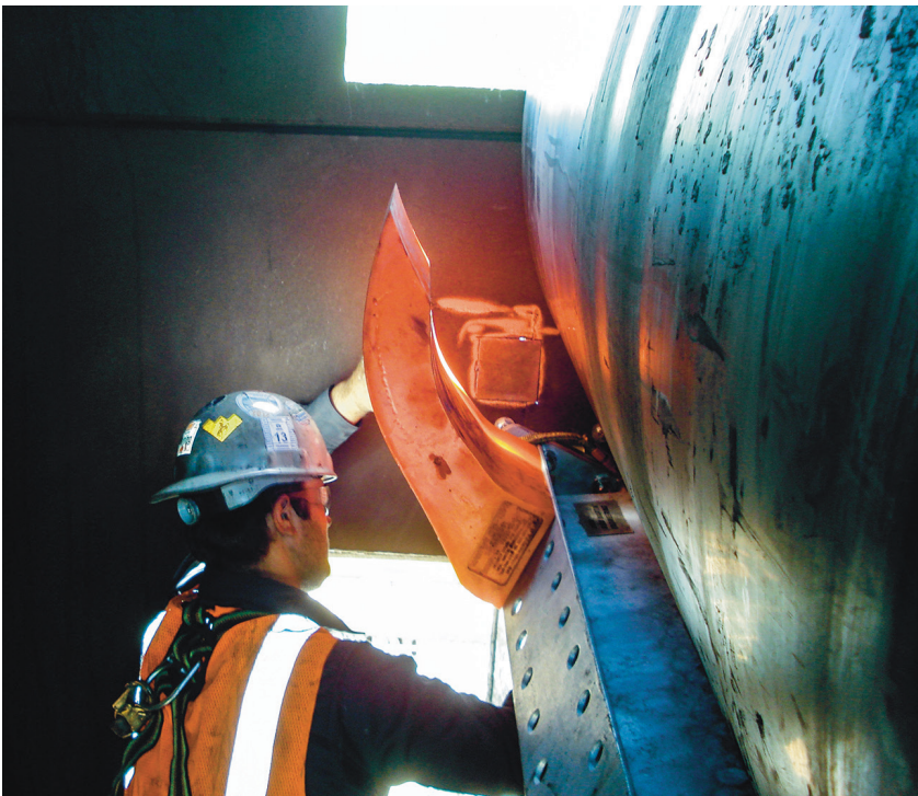
A Martin technician installs the new cleaning system, which used just two blades per belt instead of four.
