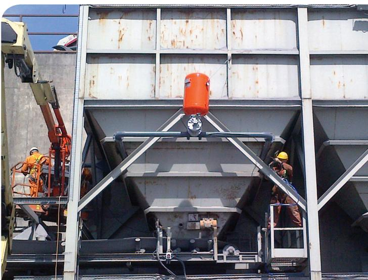
**The backside units work in tandem with a single, 150 litre cannon with a split blowpipe manifold.**
